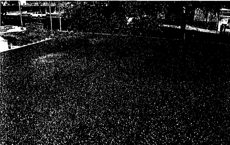
Dark areas show low spots & signs of ponding water
